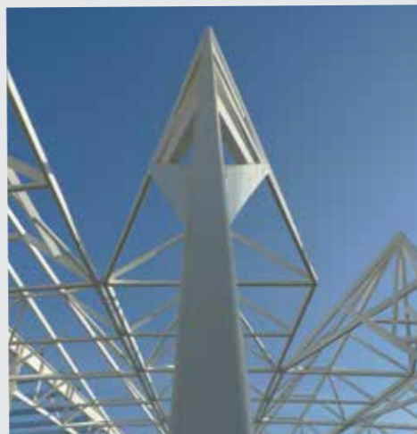
Construction of the roof of Mleiha's Visitors Centre
