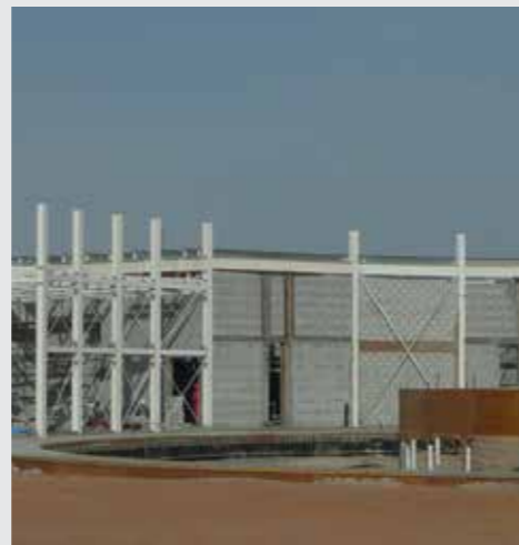
Construction of Mleiha's Visitors Centre
